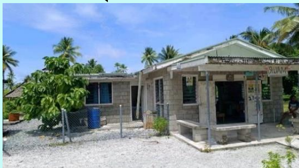
Figure 8 An outer island Health Center with an installed Starlink satellite (black arrow) and solar panels, June 2024 5 .
